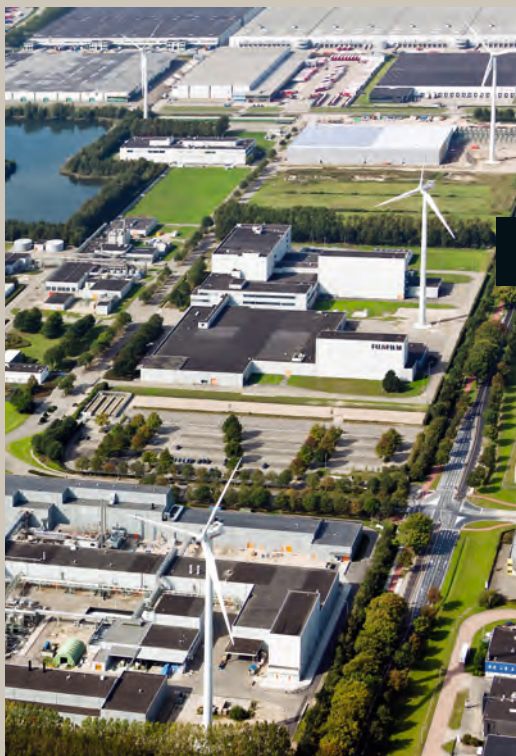
Wind turbines at the Tilburg factory provides 20% of the site's electricity needs. Photo Fujifilm.
